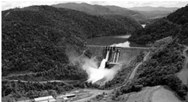
Figure XVIII: Balambano Hydroelectric Plant
