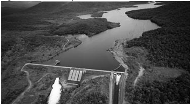
Figure XVII: Larona Hydroelectric Plant
